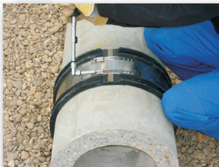
E. Assemble shear band and tighten clamps to recommended torque, see product label
